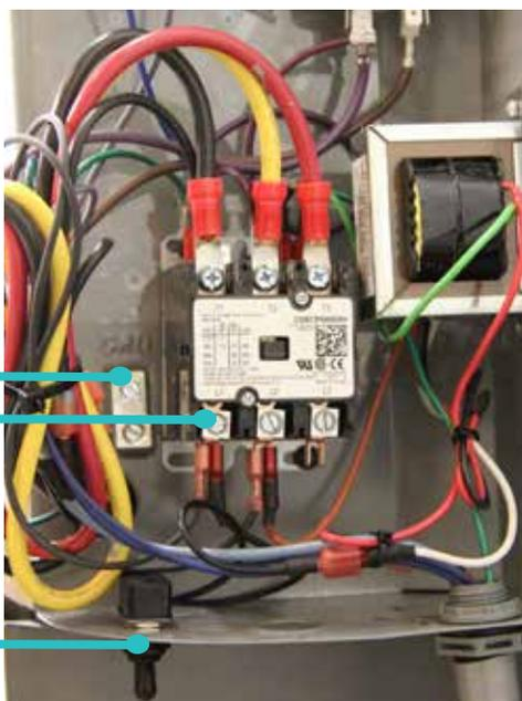
**NOTE:** If the compressor makes an unusual noise after applying 3-Phase power (10-ton 480V), the power wiring has been installed backwards. Shut the unit off immediately, shut the electric supply off at the breaker, and reverse any 2 of the 3 line conductor wires.
