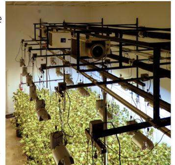
Because these units consist of multiple pieces of equipment and 99% of the indoor equipment is hung from the ceiling, having a large space dedicated entirely to climate control indoors is unnecessary. The use of multiple fan coils also ensures more homogenized air due to distributed, ductless airflow.
