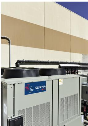
precise temperature in a water/glycol mix that is then pumped around the building to fan coil units (FCUs) of varying sizes, controlled by a simple wall thermostat or control unit with on/off control. Here, warm/moist room air is circulated over the coils, transferring heat and humidity from inside the room to condensate in the unit drain pan
